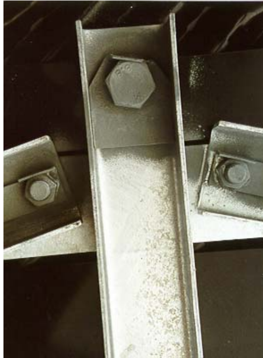
Figure 10 Use of positive locking plates on nuts and bolts
